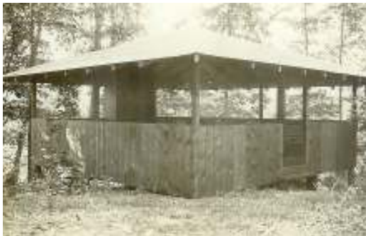
One of the three old Eagle's nest cabins
