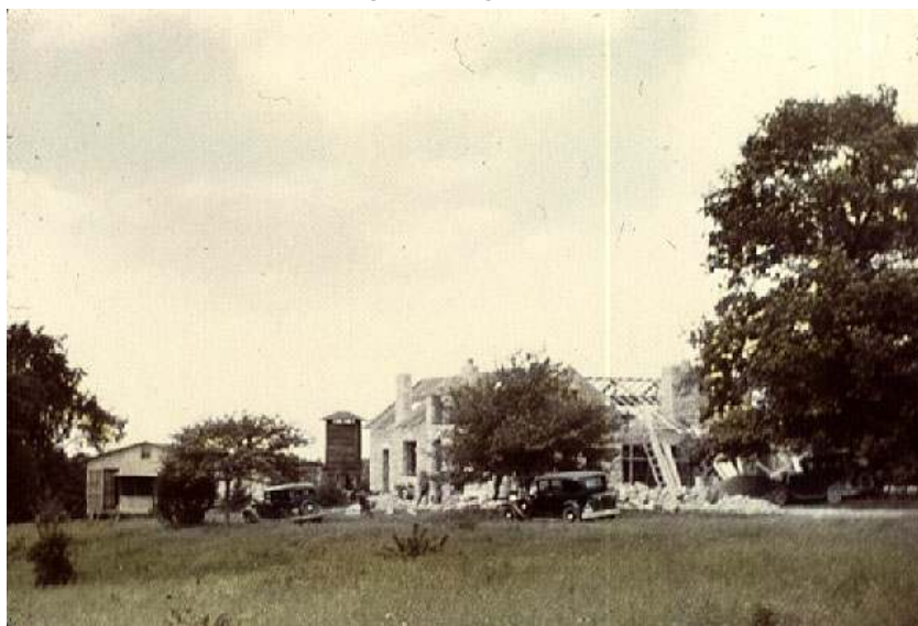
The Great Oak (far right) overlooks the construction of Eastman Lodge in 1935
