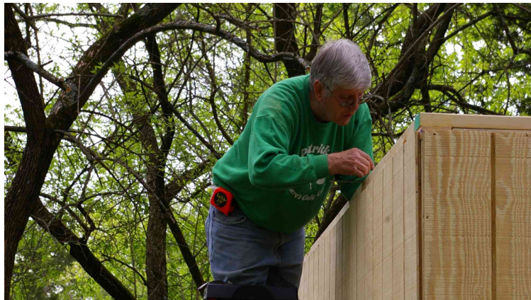
Mike Hausch works on the Vending Center construction
