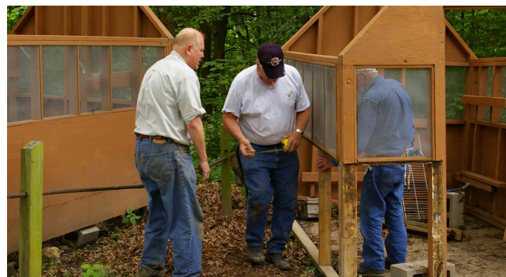
Steve Baker, Bill Ell, and Ron Keller repair a tent cabin
